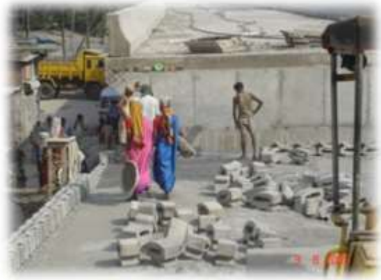
Fig. 8: Manual Handling of Blocks
