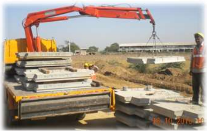
Fig. 11: Mechanical Handling of Panels
