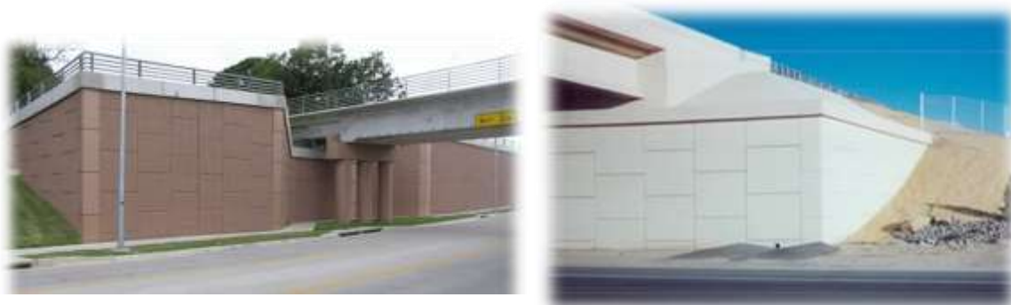
Fig. 17: Hybrid Abutment and Pure Load Bearing Abutment
