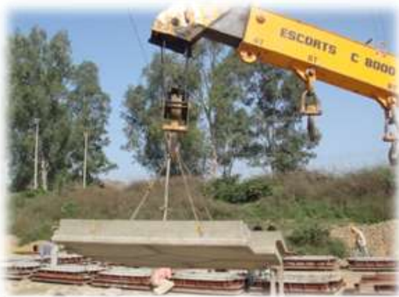
Fig. 11: Mechanical Handling of Panels
