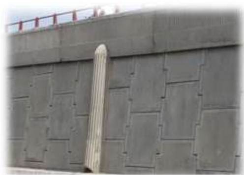
Fig. 18: Drain Pipe covered with precast pieces of similar finish
