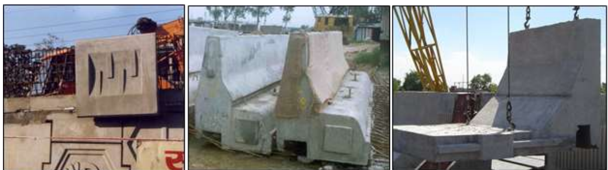
Fig. 21: Precast Crash Barrier construction: various options
