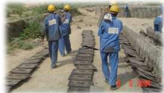
Fig. 9: Manual Handling of Blocks
