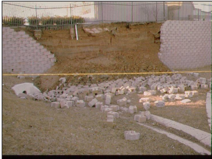
Photo 3 and 4: Two Cases of Modular Block Separation
