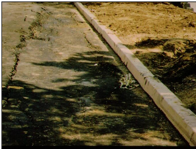
Photo 8, 9 and 10: Case of Negative Batter Development
