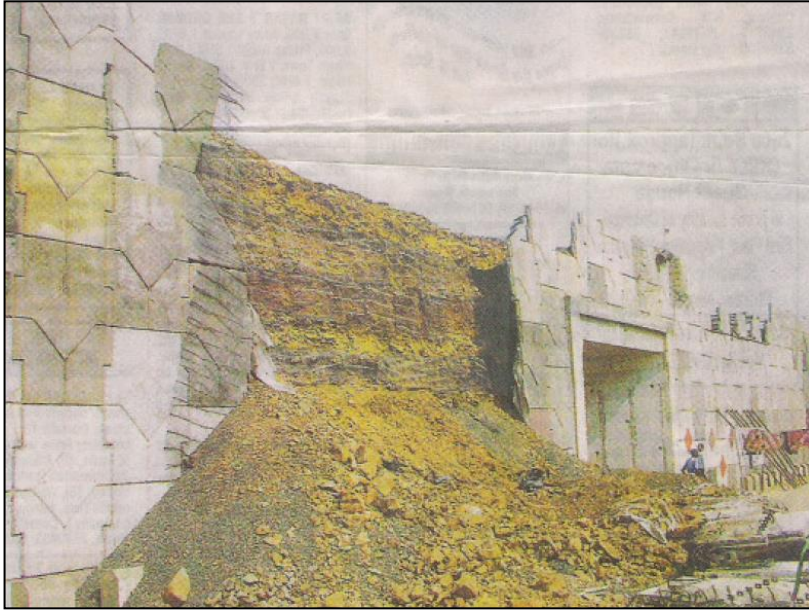
Photo 3 and 4: Two Cases of Modular Block Separation
